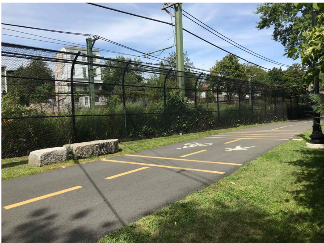
VIEW LOOKING NORTHEAST ON EAST BOSTON GREENWAY CONNECTOR
